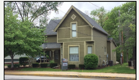
Below: 218 N. State Street, Greenfield—Pre-demolition.
