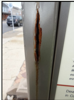
Frame damage at the Center-ville panel.
