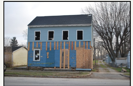
Log home with siding being removed. If a solution to relocate is not found the building is faced with demolition.
